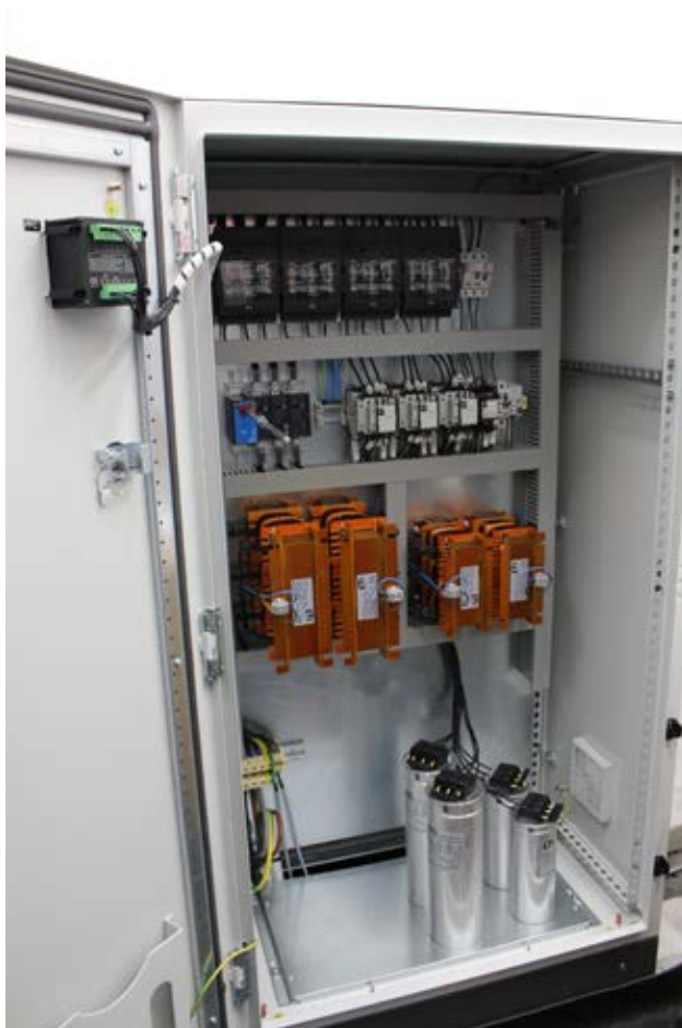
Automatic Power Factor Correction Banks
